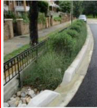
Curb extension bioretention
